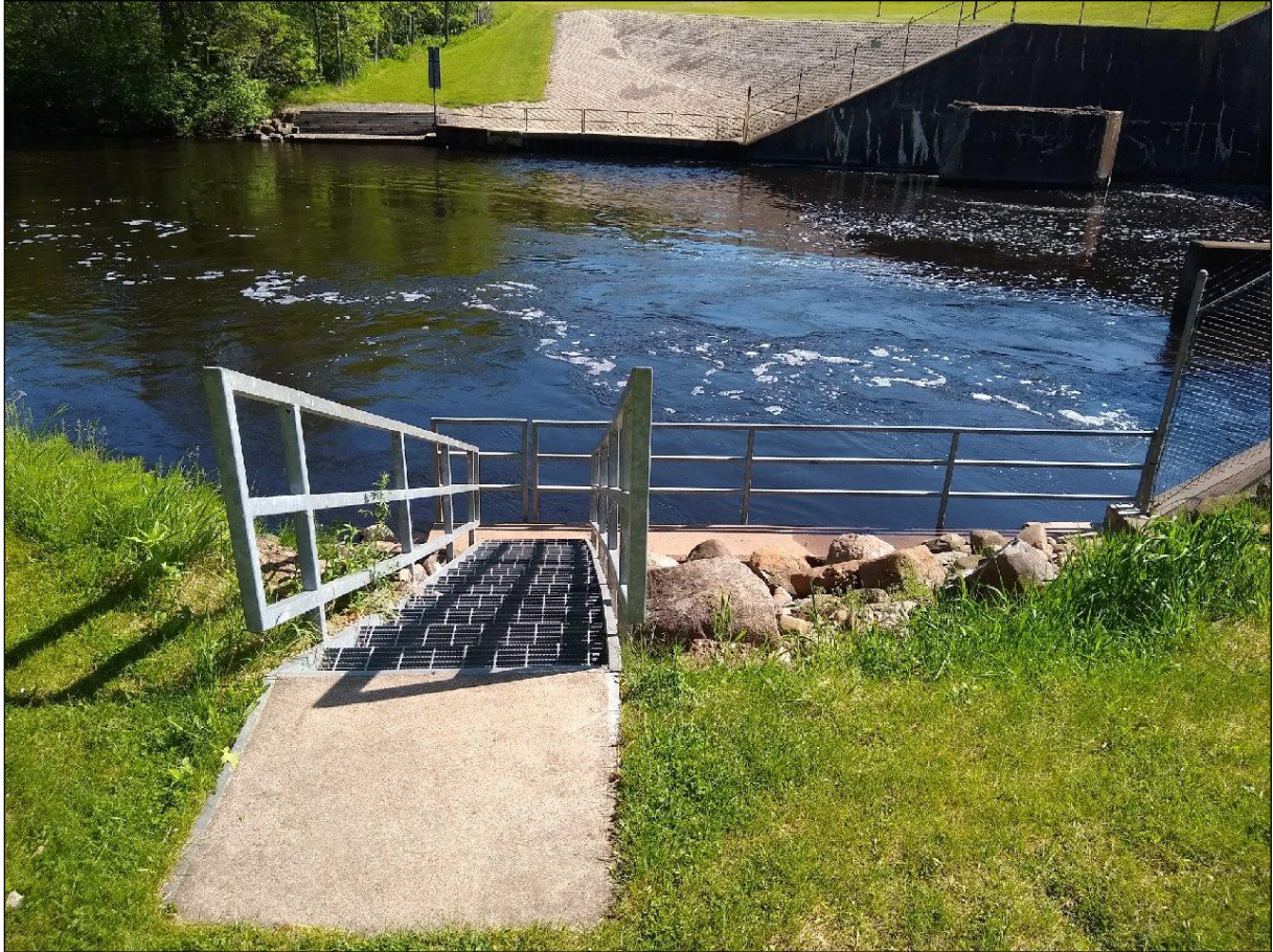
Figure 4.8.2.6-1: South Tailwater Access Stairway and Fishing Platform
