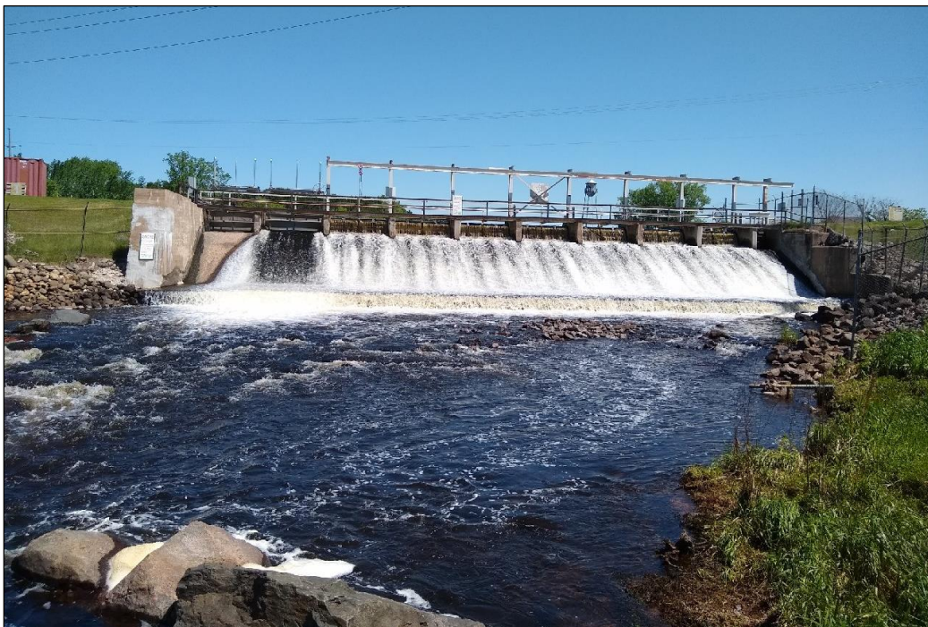
Figure 4.9.1.1-3: Hayward Project Spillway
