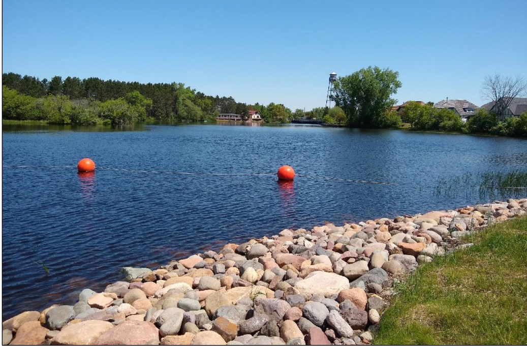
Figure 4.9.1.1-2: View Upstream of the Hayward Dam
